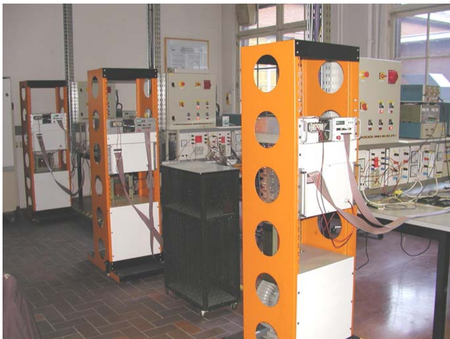
Figure: Practical setup of Herakles platform with 3 power electronic converters, interconnected via a TCP/IP based info'structure.
